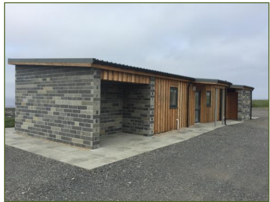
Surf Support Building at Thurso East
