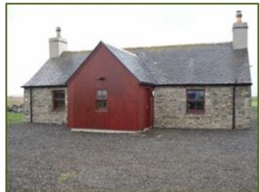
Newton Hill Woodland Community Cottage Shelter
